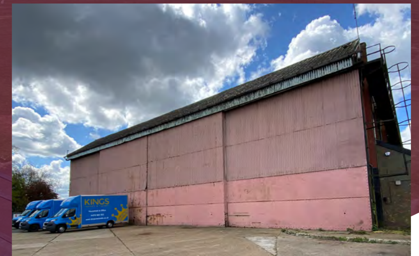
Hangar 1 - Bat Roost Potential
