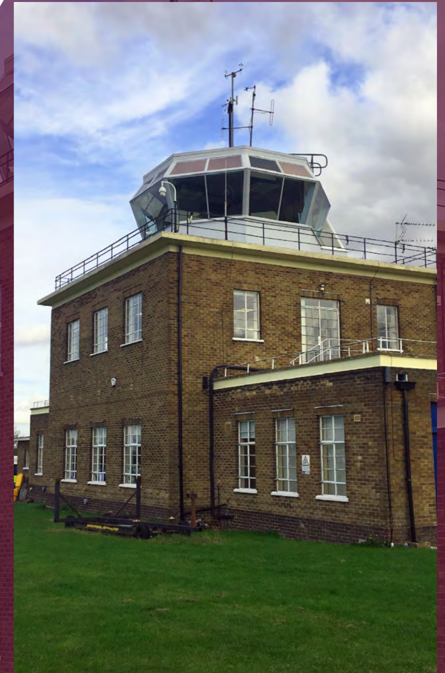
North Weald Airfield Control Tower
