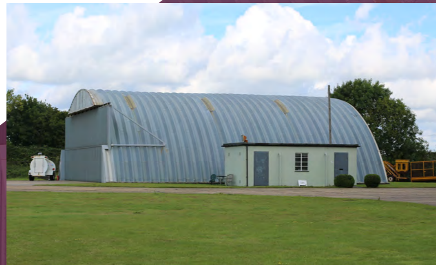
Existing hanger building located airside
