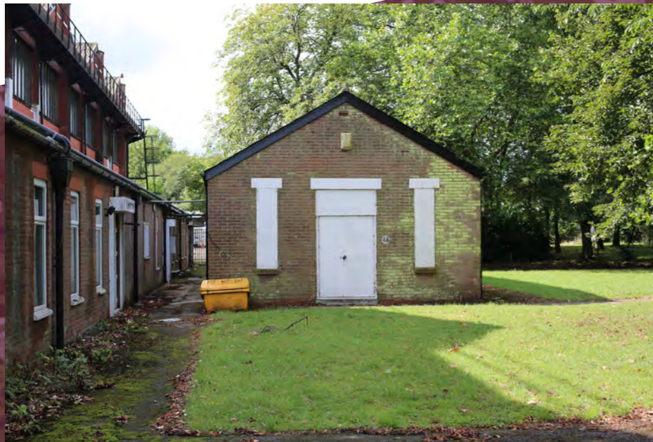
Group of trees located to the north side of Hangar 1
